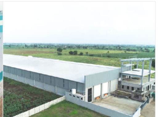
CREDENCE SOLAR PANELS PVT. LTD. - RAJKOT
