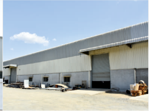
DEEPJYOT ENGINEERS PVT LTD - RAJKOT
